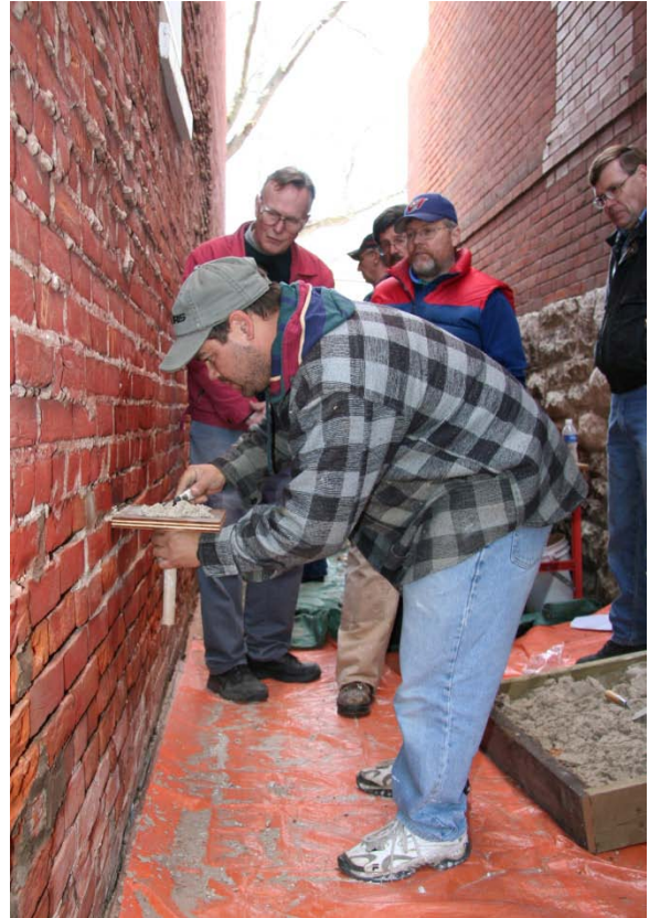
Building brick repointing workshop
