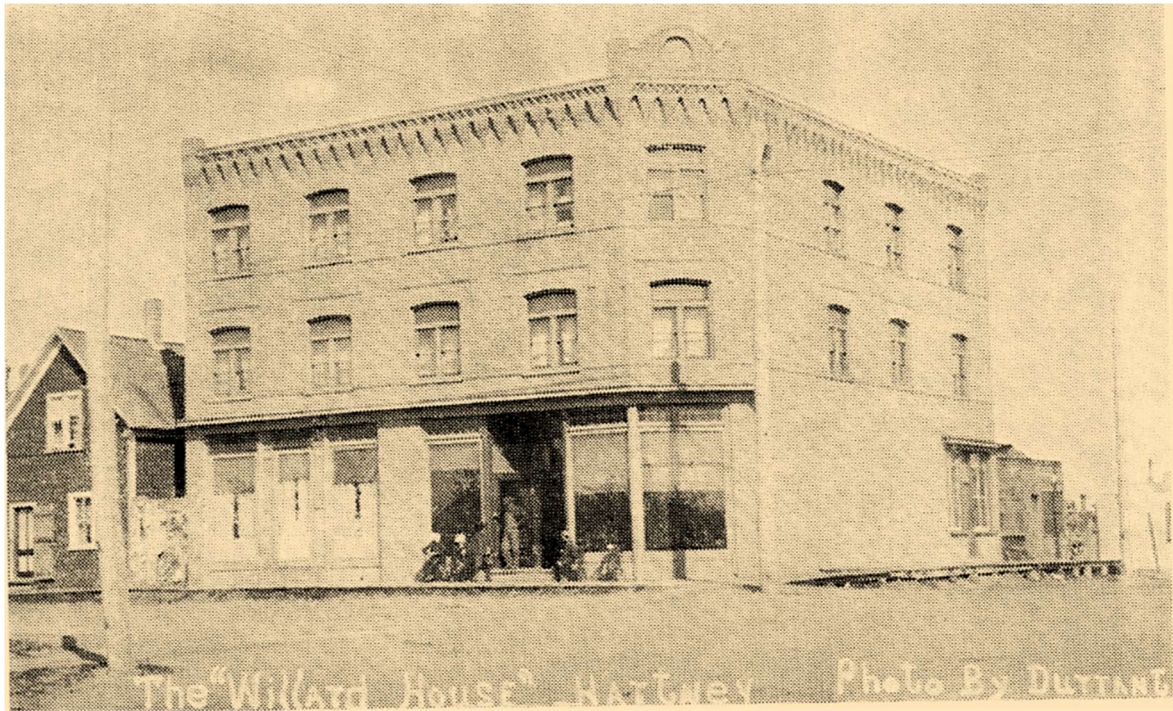
The Willard House, seen in 1908, was actually built in 1891 for William Hopkins.
