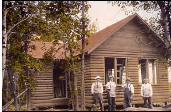
Complete Summer Cottage Or Shooting Lodge Built By North American Lumber And Supply Company in Transcona, Manitoba. It Was Sold For $395.00 (Knocked Down). - 1934. (Western Canada Pictorial Index)
