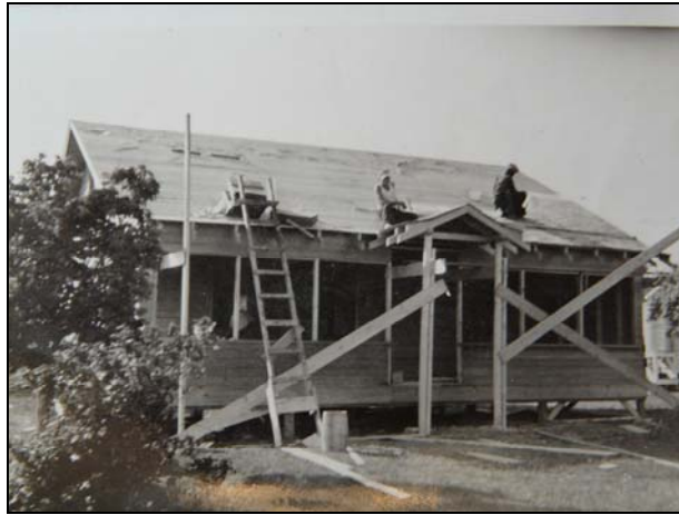
Construction of Pam Pollard's cottage – 1928 or 1929
