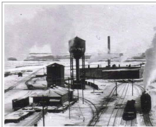
Image 6: The Roundhouse, built in 1908 and re-built in 1918. The standard service centre found at divisional points on major rail lines. With a turntable for turning the steam engines around after service.
