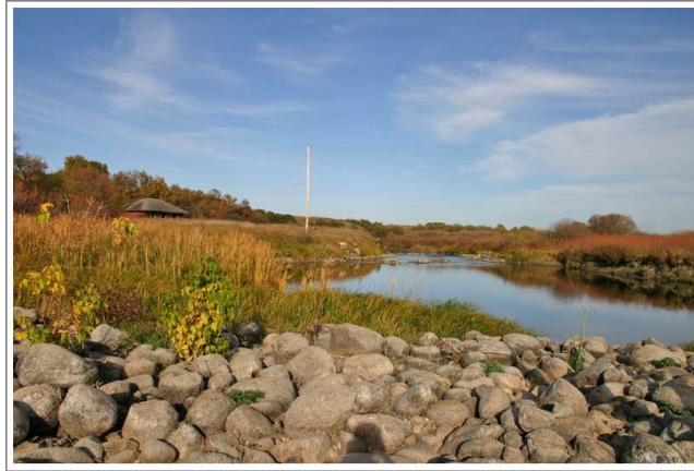
Image 14: Former site of CPR. Dam, now washing away.
