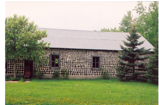
Franz Stackwall Shed. 15137 Lake Forest Road. Monica Lynn Wood and Thomas Arthur Lomeda currently own this interesting example of 1940s regional construction experiments, called stackwall.
