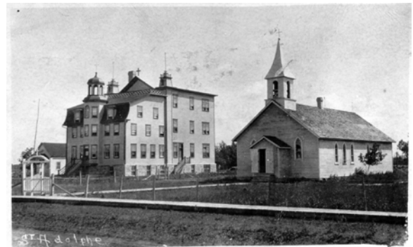
An archival image (in this case of Ste. Adolphe Church and Convent) can help walking tour readers imagine what a building once looked like, or, if it has been lost, what the site once looked like.
