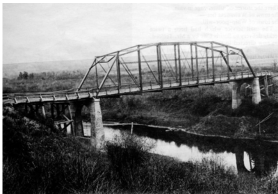
"Black" South Traffic Bridge. Built in 1908 and still in use.
