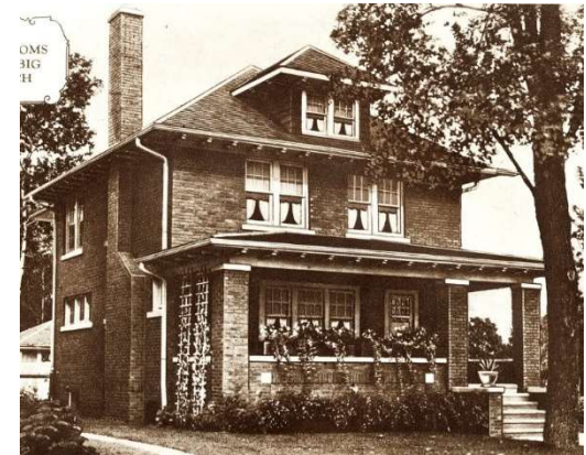
An illustration from a 1920s Sears catalogue shows a typical American Four-square, a very popular house design seen throughout Manitoba from about 1890 to 1920. Such a house would have required about 15,000 bricks in its construction. (WikiCommons)
