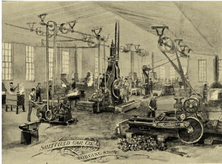
This rendering, of the Sheffield (England) Car Company has been featured to more clearly show the use of drive shafts, assembly lines and connections by belts to the sheaves on the line and thence to the individual pieces of machinery.
