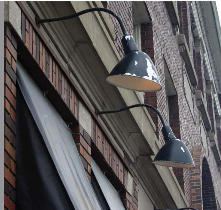
Note the shape and angle of the gooseneck light's projecting arm: it comes straight out from the building, parallel to the ground, then curves up before curving back down towards the sign it is intended to light. This shape allows for the clearance of other architectural features.
