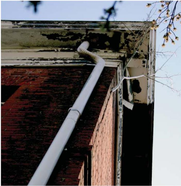
Note the deterioration of the painted metal cornice near the downspout. Water has damaged the finish, as well as some of the mortar joints in the masonry. In order to fix the paint, the downspout connection should be checked to ensure that a new painted finish will not quickly deteriorate because of the same underlying problem.
