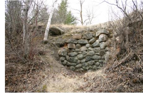
The LIME KILN SITE is an important, and now rare, reminder of the kind of pioneer industrial and manufacturing activity required in the construction of buildings. It was here that the lime used for the production of mortar was produced by burning limestone (which is abundant in Birtle); the mortar produced here was used in the construction of nearly every foundation in town and in all the masonry buildings as well.
